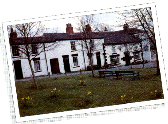
Properties adjacent to the Great North Road in the centre of Aberford
