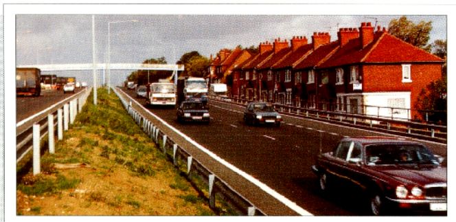
Looking north on the existing road at Skellow
